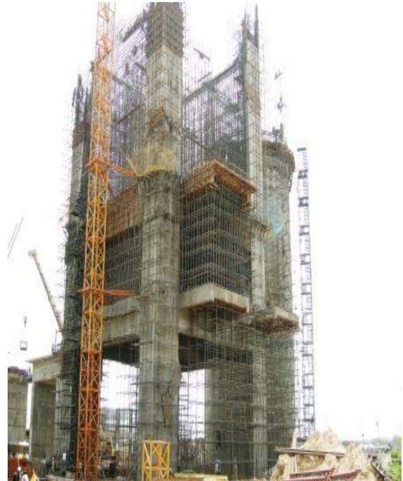
Ariyalur, TN Cement Plant
